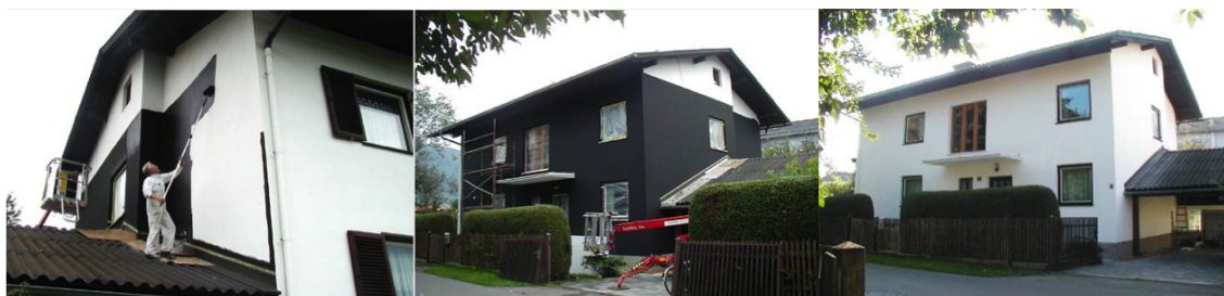
Figure 3.7: Some of the applications where carbon conductive paint is coated (adapted from [46]). From the Figure it can be observed that a man started painting a house with carbon paint (left most and middle figure) and in order to protect the carbon paint, it is top coated with a white paint (right most).
