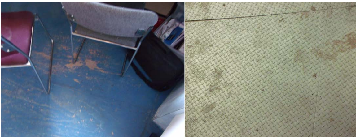
Figure 4: MDRS interior deck-cover. Upper level wood (left) and lower level metal (right).
