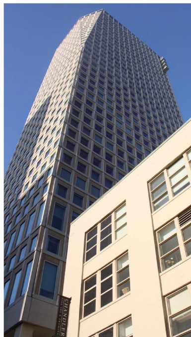
Fig. 11. Skyscraper facade in San Francisco city center. Different window frames are present on the upper and lower parts of the facade (lower part: 15 floors with 15 windows; upper part: 17 floors with window number decreasing from 15 to 11). Moritz Rexer, TUM.
