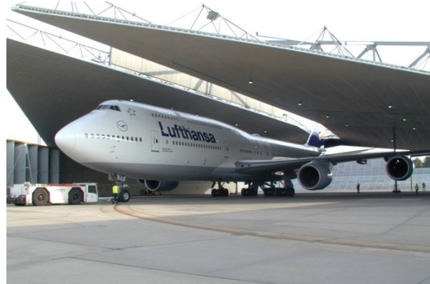
Figure 3: Sound-attenuating hangar at Hamburg Airport (left), a B747-800 inside the hangar (right) [3]
