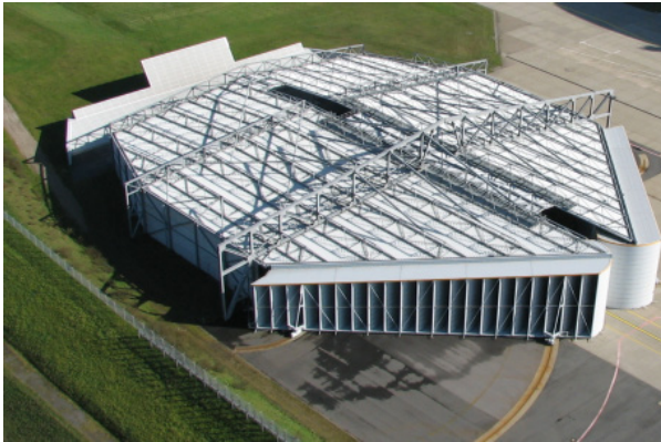
Figure 3: Sound-attenuating hangar at Hamburg Airport (left), a B747-800 inside the hangar (right) [3]
