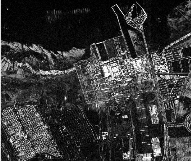
Fig. 5: Oil pier in Kuwait: industrial facilities (Latitude 29.35° / longitude 47.76°; May 09, 2013)
