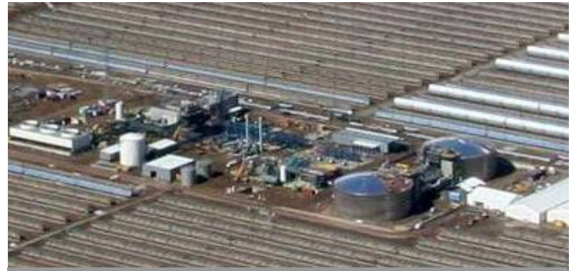
1000 MWh molten salt storage at Andasol plant
