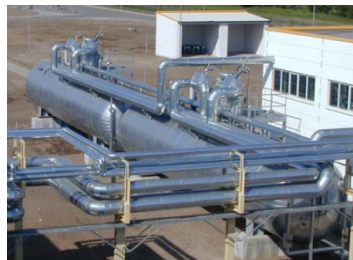
Sliding pressure storage for gas concrete manufacturing
