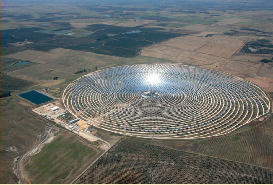
A typical CSP plant
