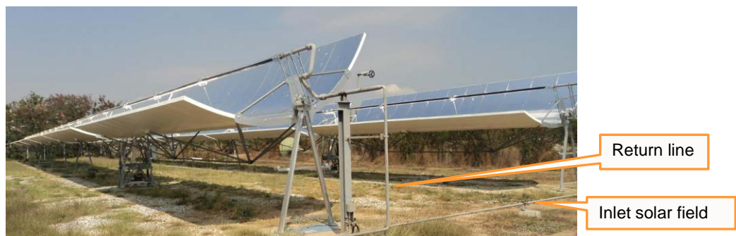
Fig. 1. Solar field with SL4600 collectors
