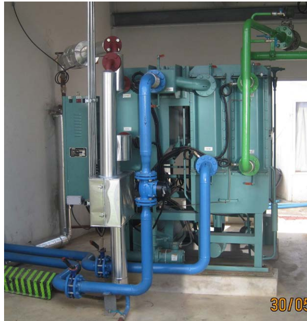
Fig. 5. Absorption chiller
