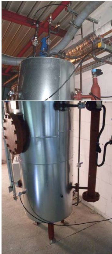
Fig. 4: Steam drum with level indicator at the right (left) and touch screen for control (right)
