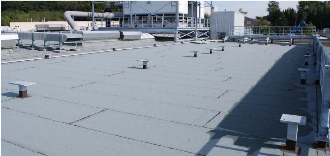
Fig. 2: Pedestals for collector pylons and drive system (before collector mounting)
