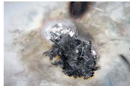
Damage by Lightning Strike
