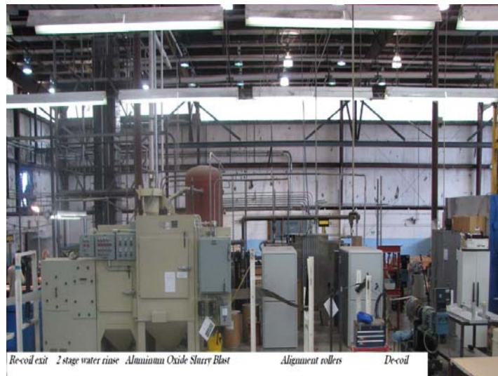
Fig. 3.4: MOD-1: slurry grit blast.
