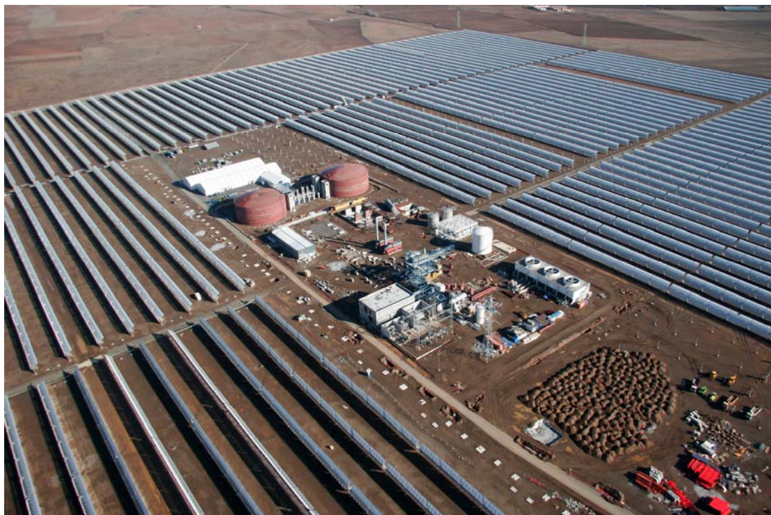
Figure 3-38: Andasol-1 parabolic trough solar field, storage tanks and power station during construction in December 2007 (Source: ACS Cobra S.A., Spain).
