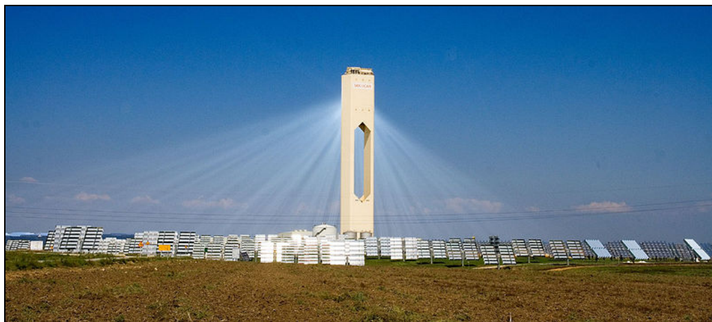
Figure 3-43: PS 10 central receiver solar tower facility near Sevilla, Spain (Abengoa Solar)
