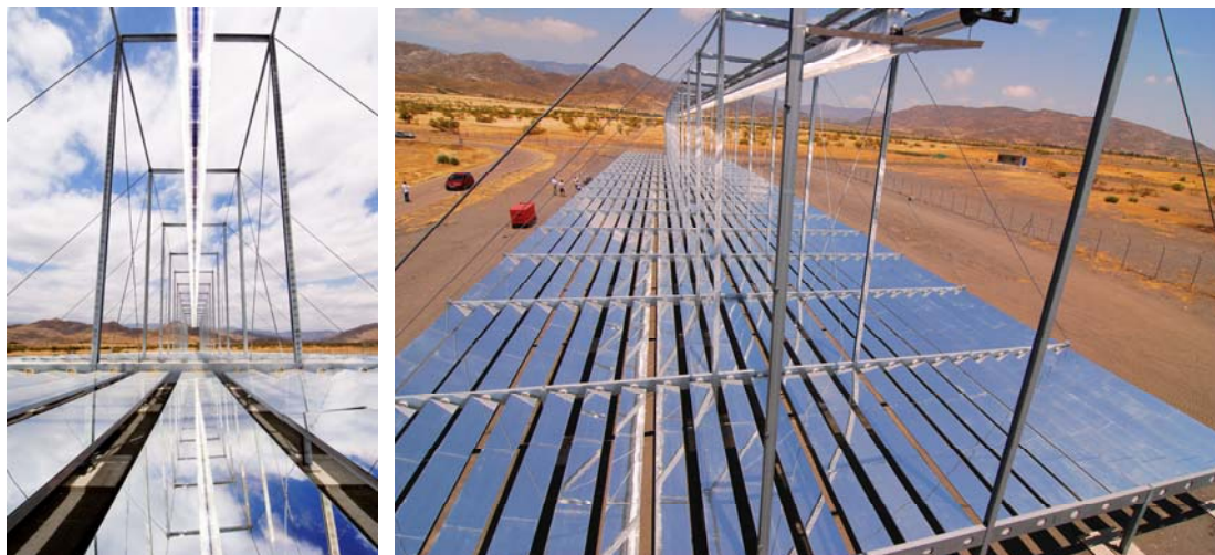
Figure 3-41: Absorber tube box (left) and linear Fresnel collector assembly (right) of the FRESDEMO project at Plataforma Solar de Almeria, Spain (Source: MAN/SPG).
