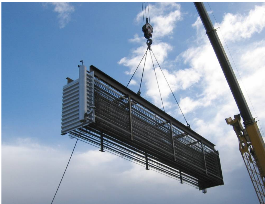
Figure 2: Lifting of the prefabricated tube register
