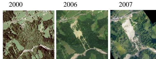
Fig 7 The slope failure in Austria in the years 2000, 2006, and 2007
