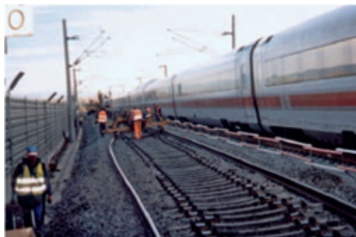
Figure 4: Fixed barrier between the track in operation and the construction site [2]
