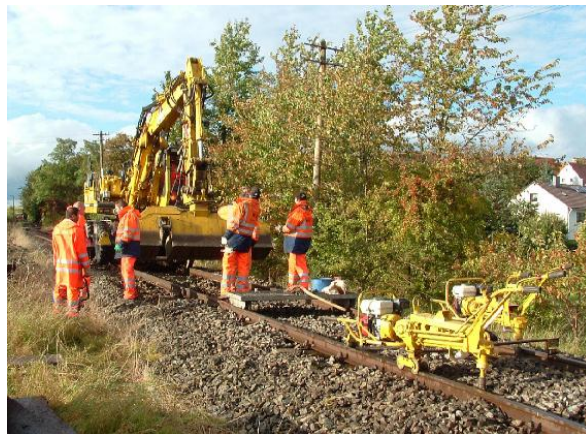
Figure 2: Working situation of gang workers on a railway construction site [1]
