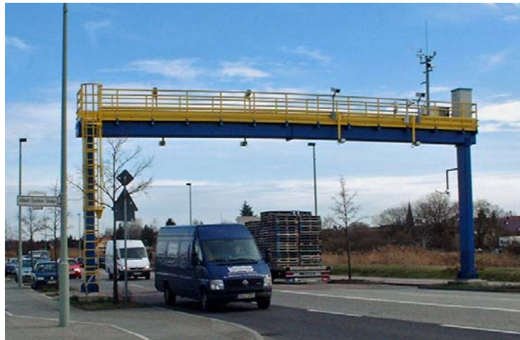
Figure 3 - Experimentation road at DLR Berlin for the system tests
