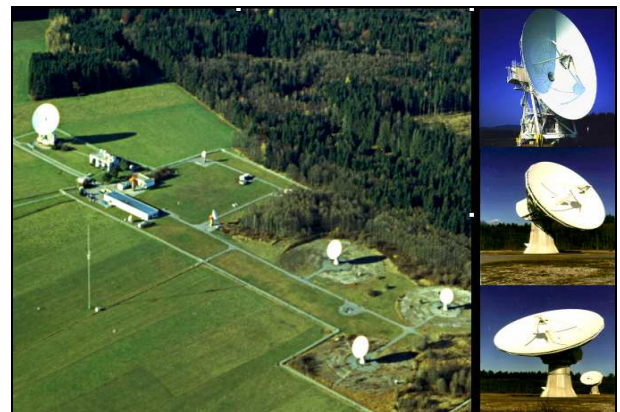
Figure 5: The ground station complex of GSOC at Weilheim. The main multimission antennas are two 15 m S-Band dishes.
