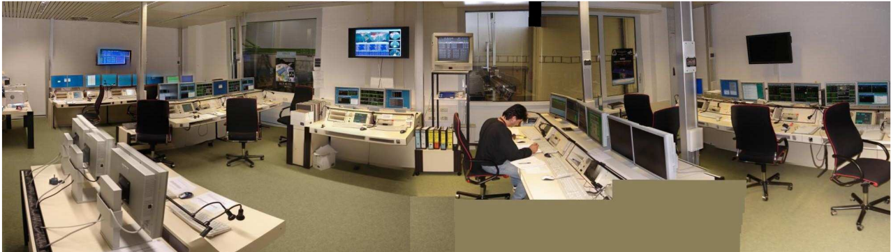
Figure 2: Panoramic view of the Multimission Control Room at GSOC. GRACE 1&2 operations are performed from the two rows of consoles in the background at the left side, CHAMP consoles are in the middle part, and BIRD consoles are in the background to the right.
