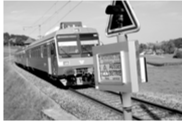
Fig.4. An innovative LX system with light signal at Emmental [4]
