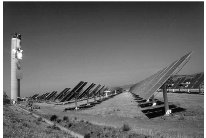
FIGURE 1: The Cesa 1 tower at the ‘Plataforma Solar de Almería’ (PSA) used as test installation for solar air receivers
