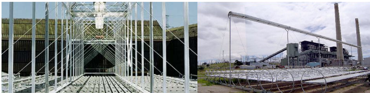
Figure 1: Prototype of the linear Fresnel collector by the Belgian company Solarmundo (left), Fresnel collector prototype by Solar, Heat and Power, Australia (right)
