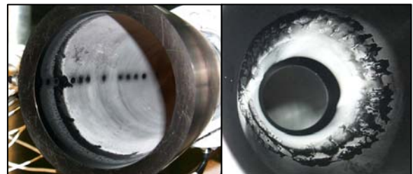
Fig. 7: “BFF” view to the nozzle
