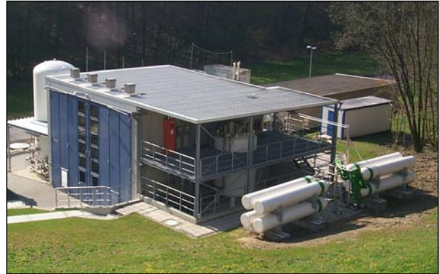
Fig. 5: P4 Steam Generator Building
