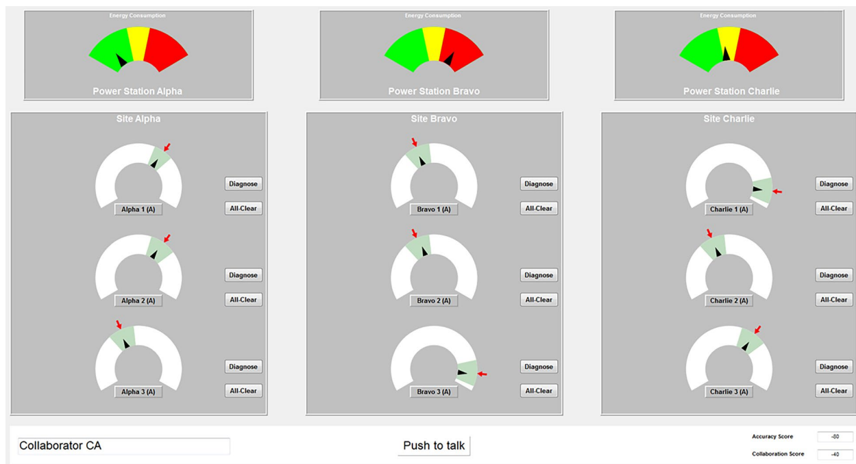
Figure 3. Monitoring screen of ConCentT containing the displays of nine production facilities and three power stations, which are distributed over three locations.
