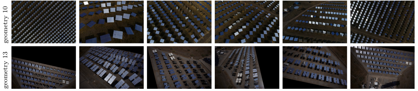
Fig. 2. Top row: Images recorded during a measurement flight over the STJ plant, showing heliostat collector geometry 10 and supplementing the evaluation in this study. Bottom row: Masked images from the measurement flight by Jessen et al. [6] at the PSA (owned and operated by CIEMAT), showing heliostat collector geometry 13 and used in the evaluation of both previous work and the present study.
