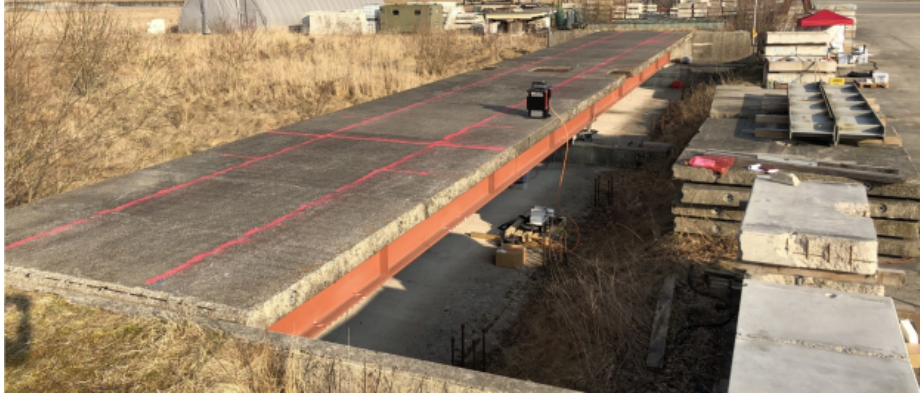
Fig. 1: Overview of the test bridge, with top deck concrete slabs clearly visible, together with part of the southern principal HEB1000 girder.
