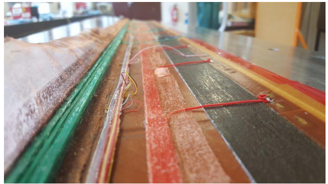
Fig. 12. Finished cabling and shielding
