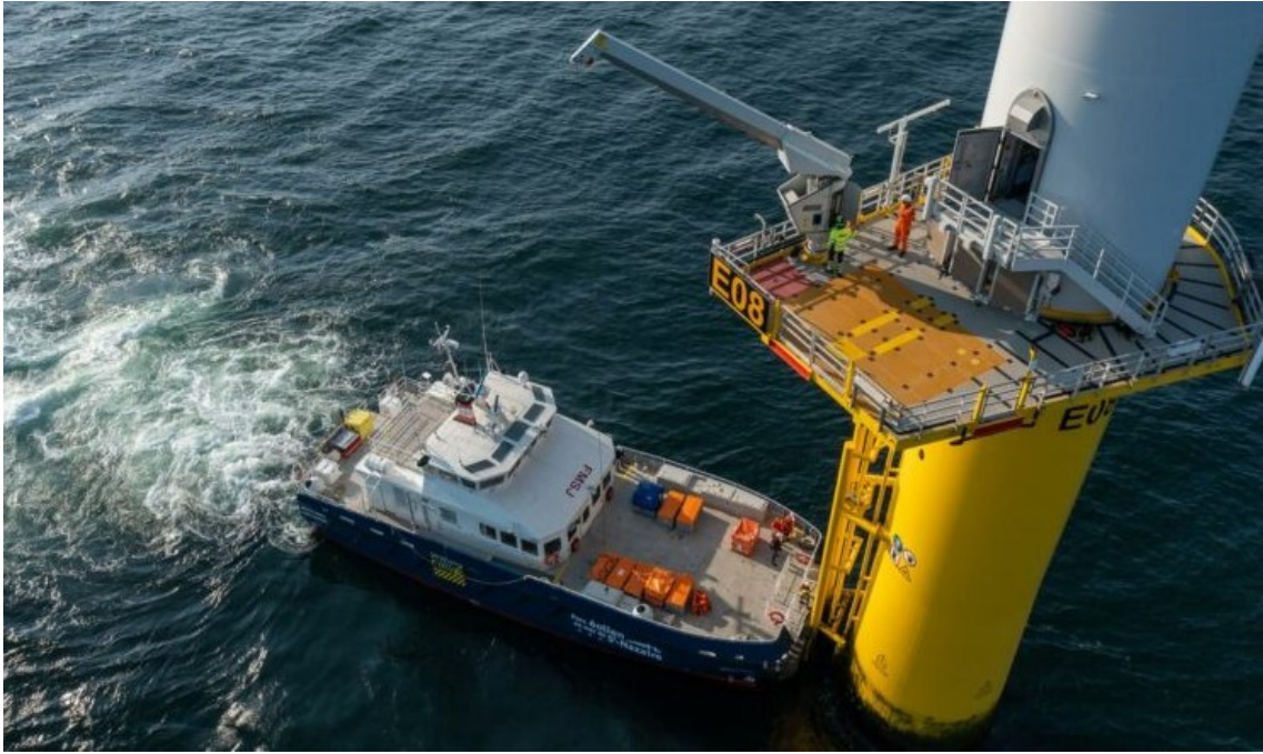
Figure 2.17: Transfer of Equipment from CTV to a Turbine's Transition Piece [109]
