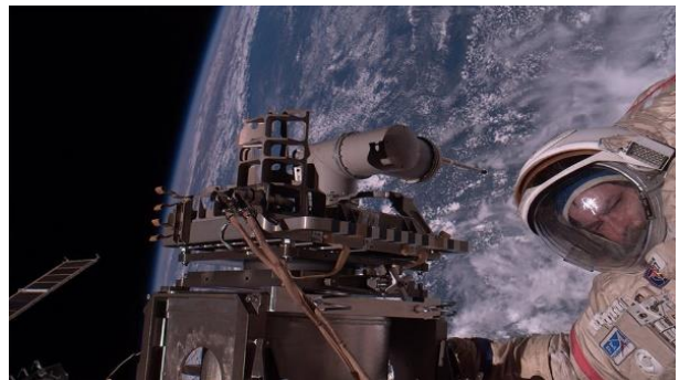
Figure 3. Mounting of the ROKVISS on the ISS. Credit: RKK-Energija.
