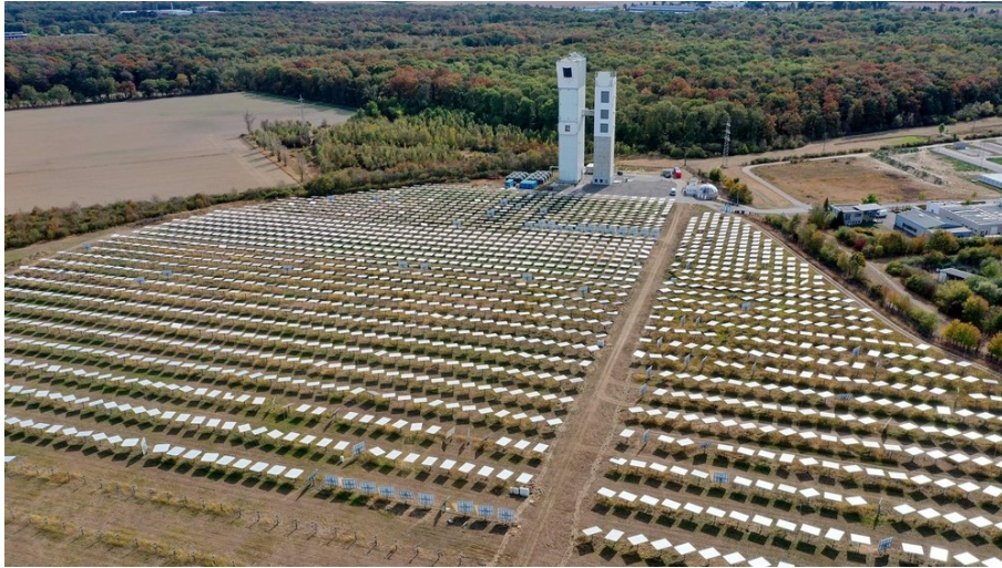
Figure 1: Over 2000 mirrors concentrate incoming sunlight onto the tips of the solar tower at Juelich, Germany. Credit: DLR, CC BY-NC-ND 3.0.
