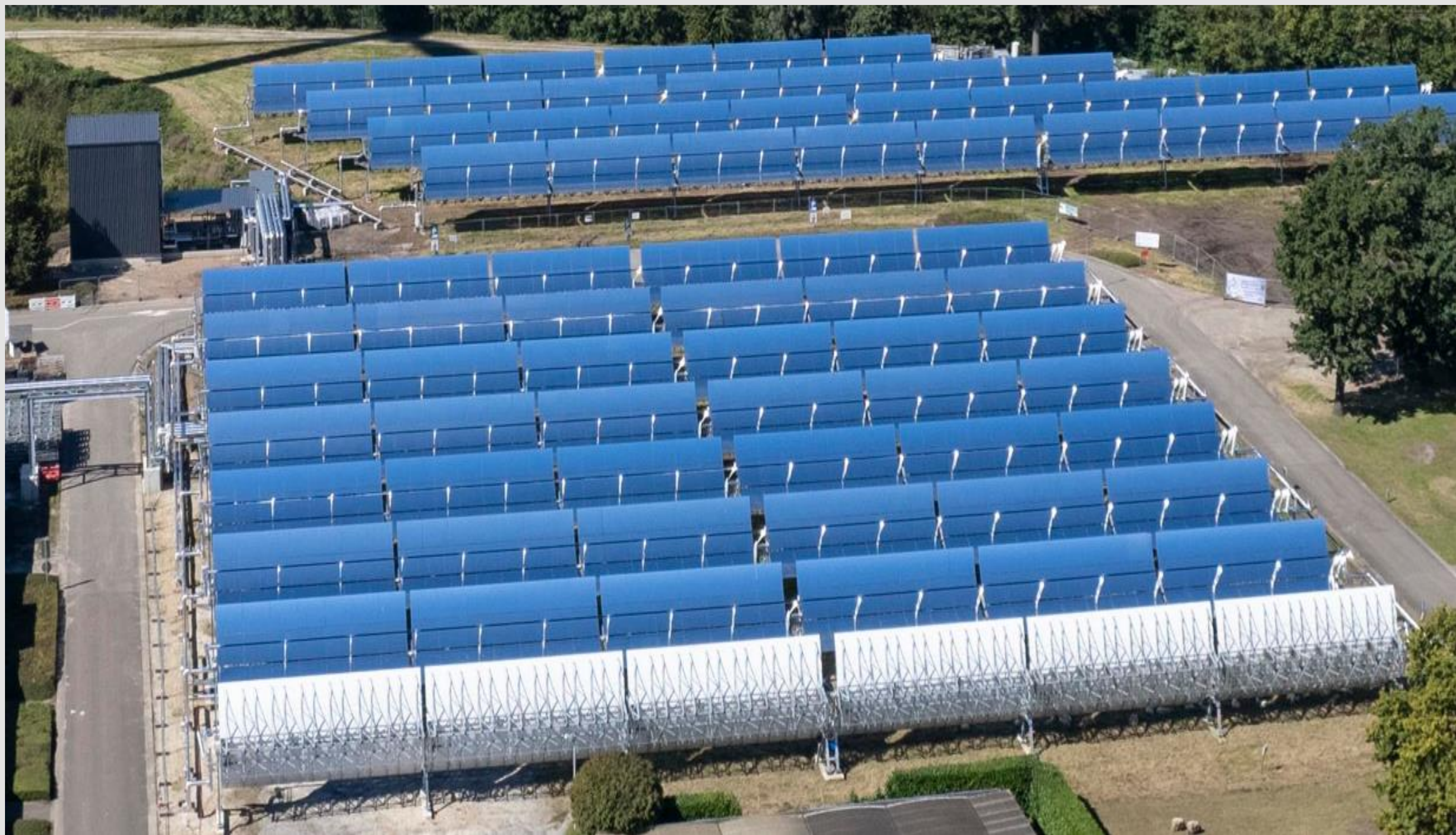
Figure 2: View of the parabolic trough field in Turnhout (photo: Avery Dennison)
