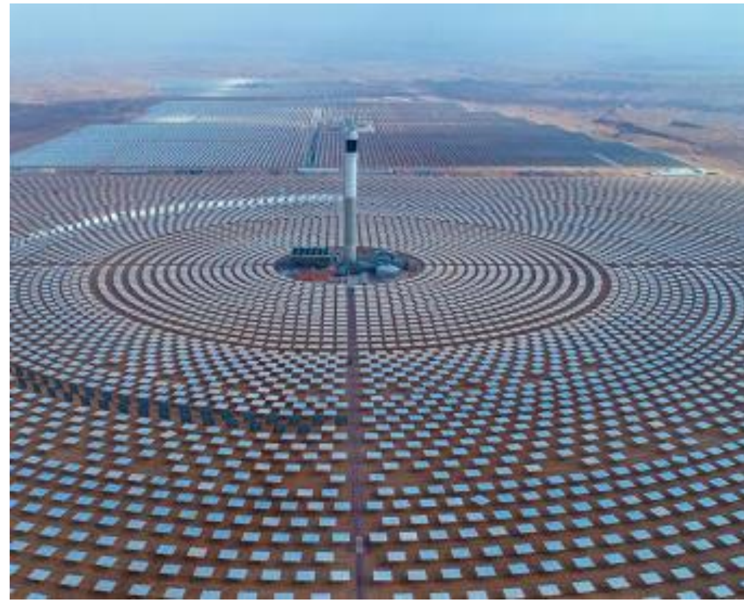
Solar tower system
