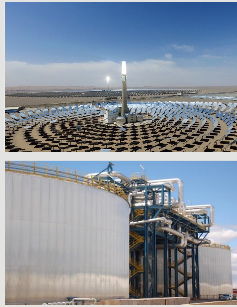
Fig.1: Top: Concentrated solar power (CSP) plant with a power tower configuration. Bottom: Molten salt storage tanks
