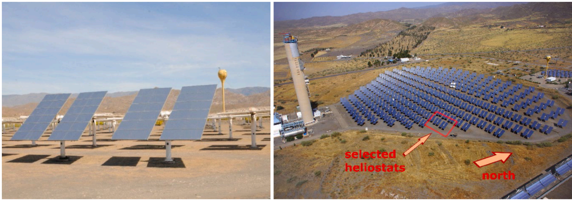
Fig. 1. The two heliostats, H18 and H20, used for the campaign during tracking (left) and the layout of the CESA1 solar field with position of heliostats (right).
