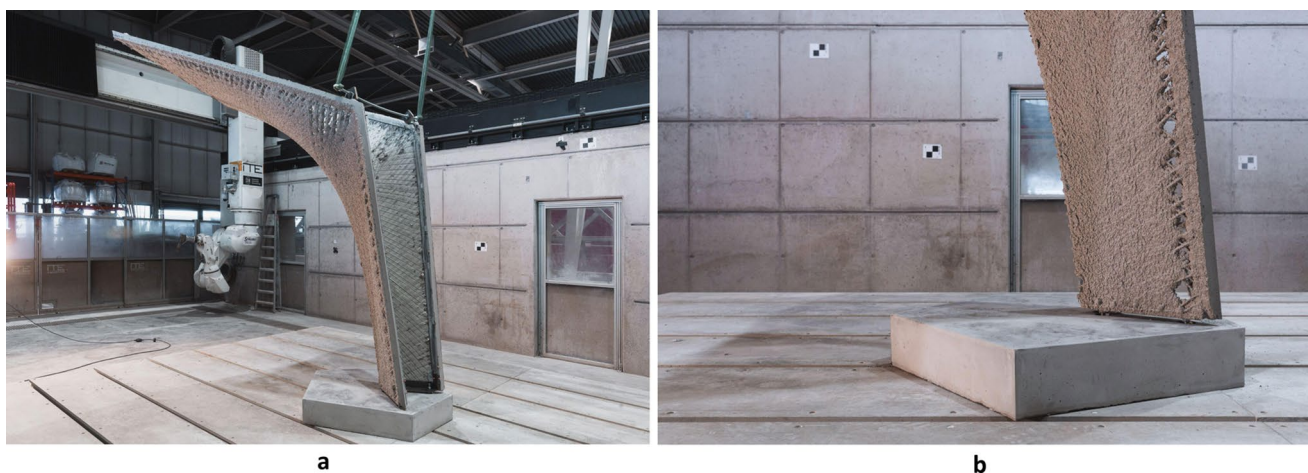
Fig. 19 Crane-assisted assembly of the pavilion segment (a) onto a pedestal (b) by means of four tailored anchor bolts
