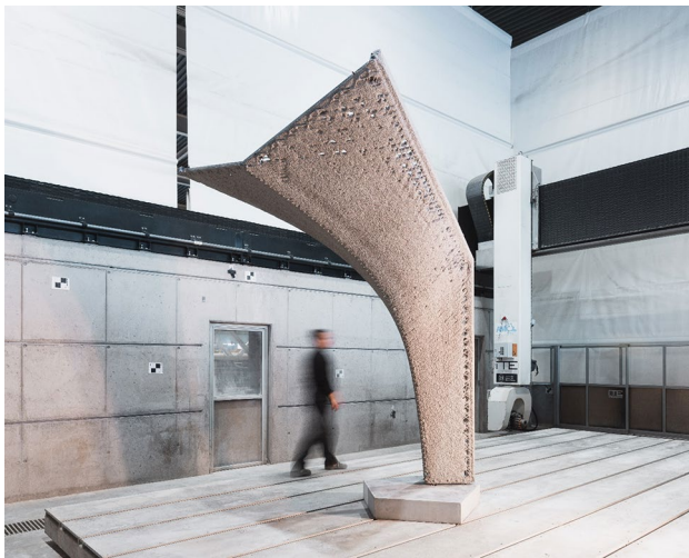
Fig. 24 The pavilion segment serves as a demonstrator for cutting-edge digital fabrication research. It highlights the potential of Robotic Fibre Winding for concrete construction, resulting in a structurally sound and visually compelling piece
