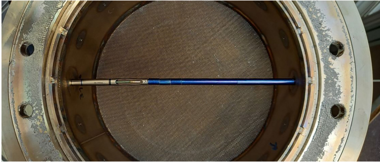
Fig. 36. Realization of probe extension using sleeves (blue, each 10 mm) from the opposite end.
