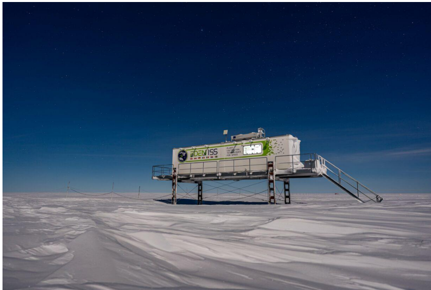
Figure 2.2.2 - EDEN ISS Mobile Test Facility [5]
