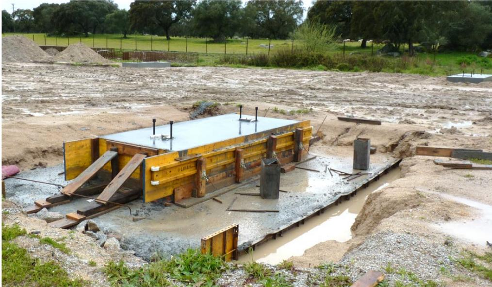
**Figure 19 – Finishing of upper foundation pedestal with second formwork & casting**
