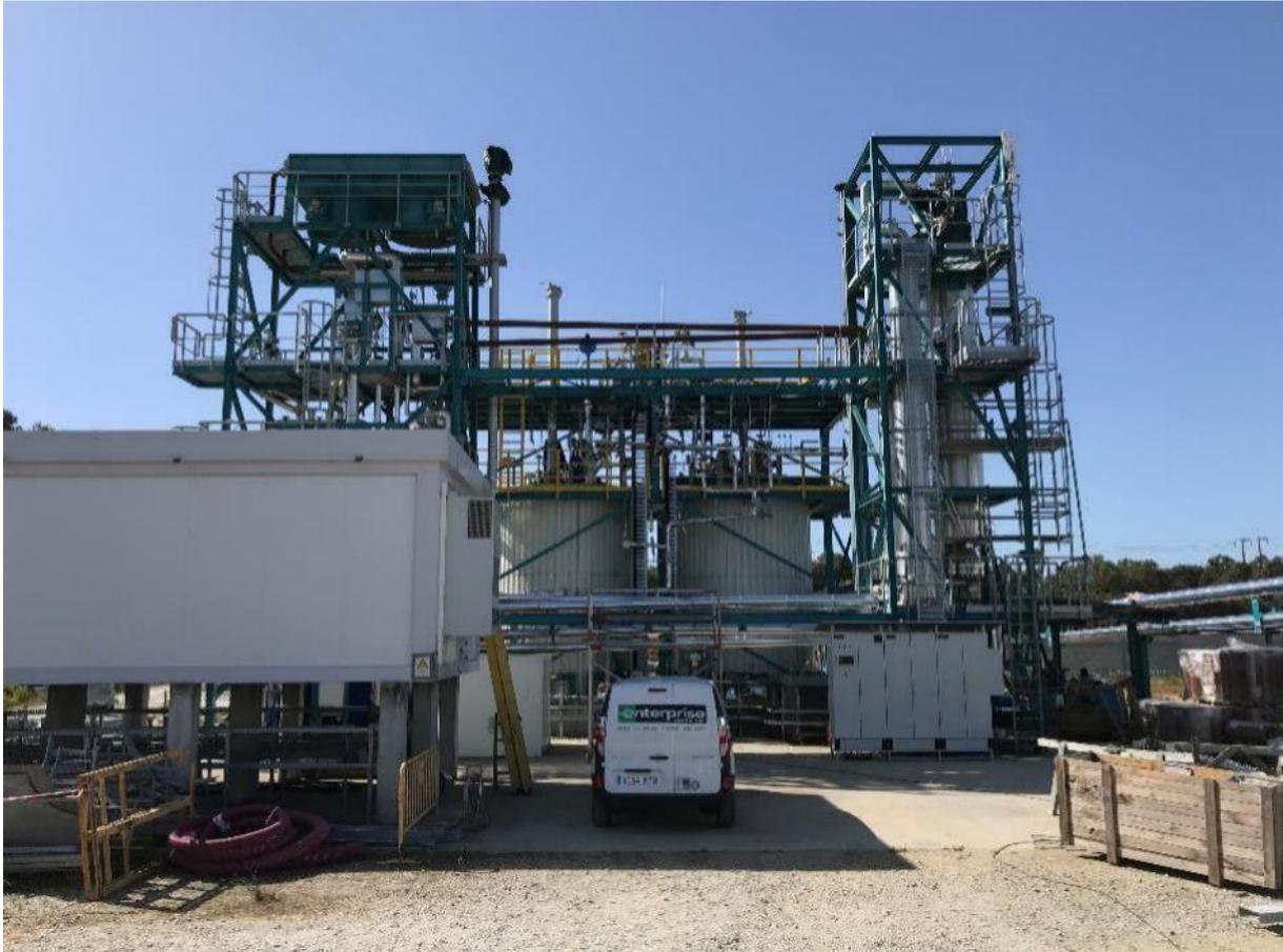
**Figure 44 Completed SGS skids.**
