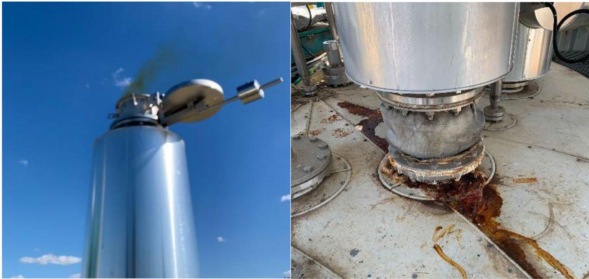
**Figure 77: NO<sub>x</sub> emissions after melting process (left), nitrite acid leakage on the compensator of the cold tanks chimney (right)**
