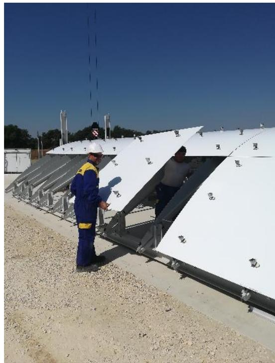
**Figure 31 - Installation of glue-pods and placing the mirrors in the mirror jig**
