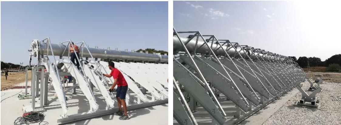
**Figure 30 – Installation of the cantilever arms in the eSteelStructure Jig**
