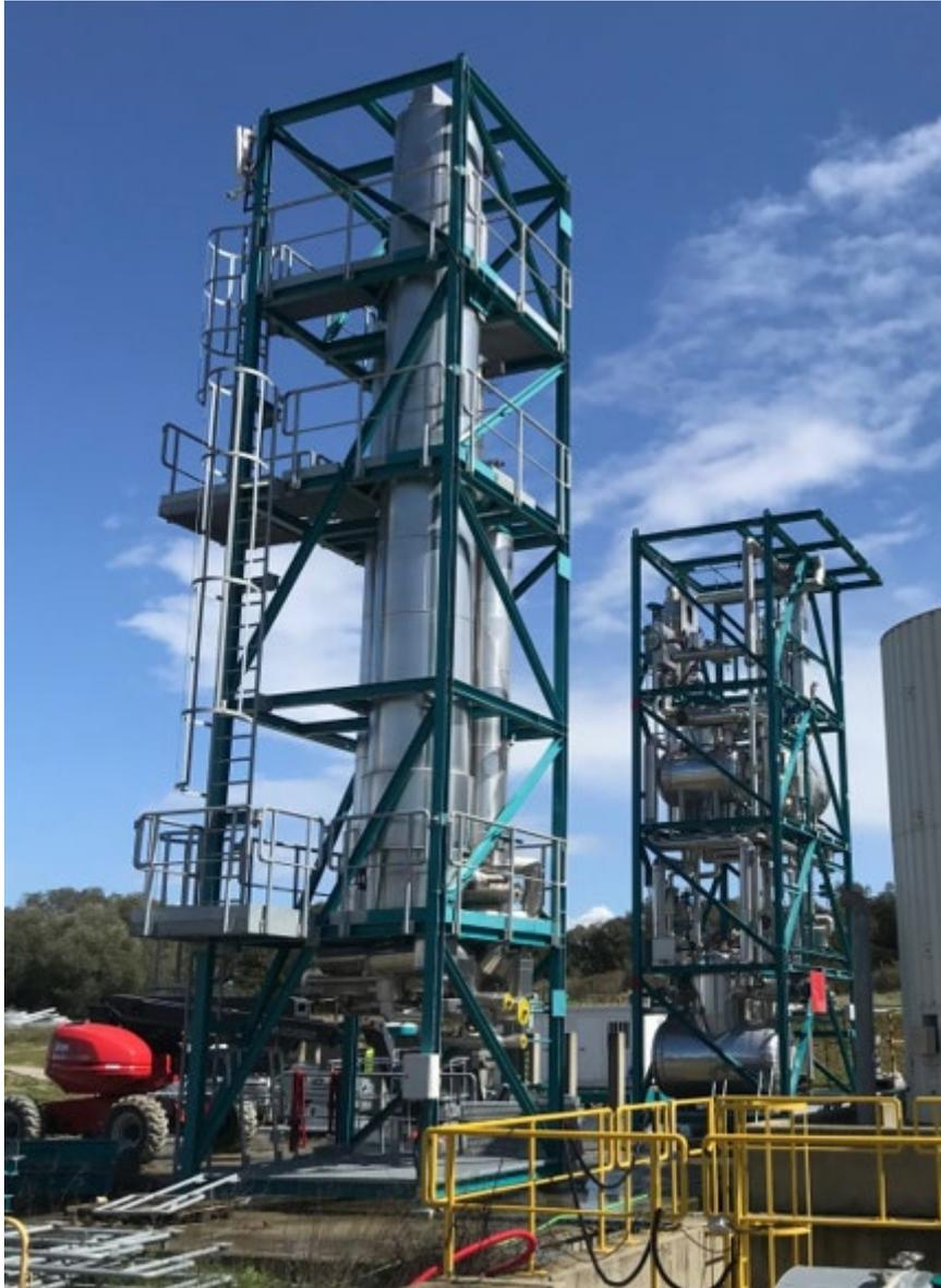
**Figure 43 Installation of grating, ladders and platforms on pre-fabricated SGS skids**
