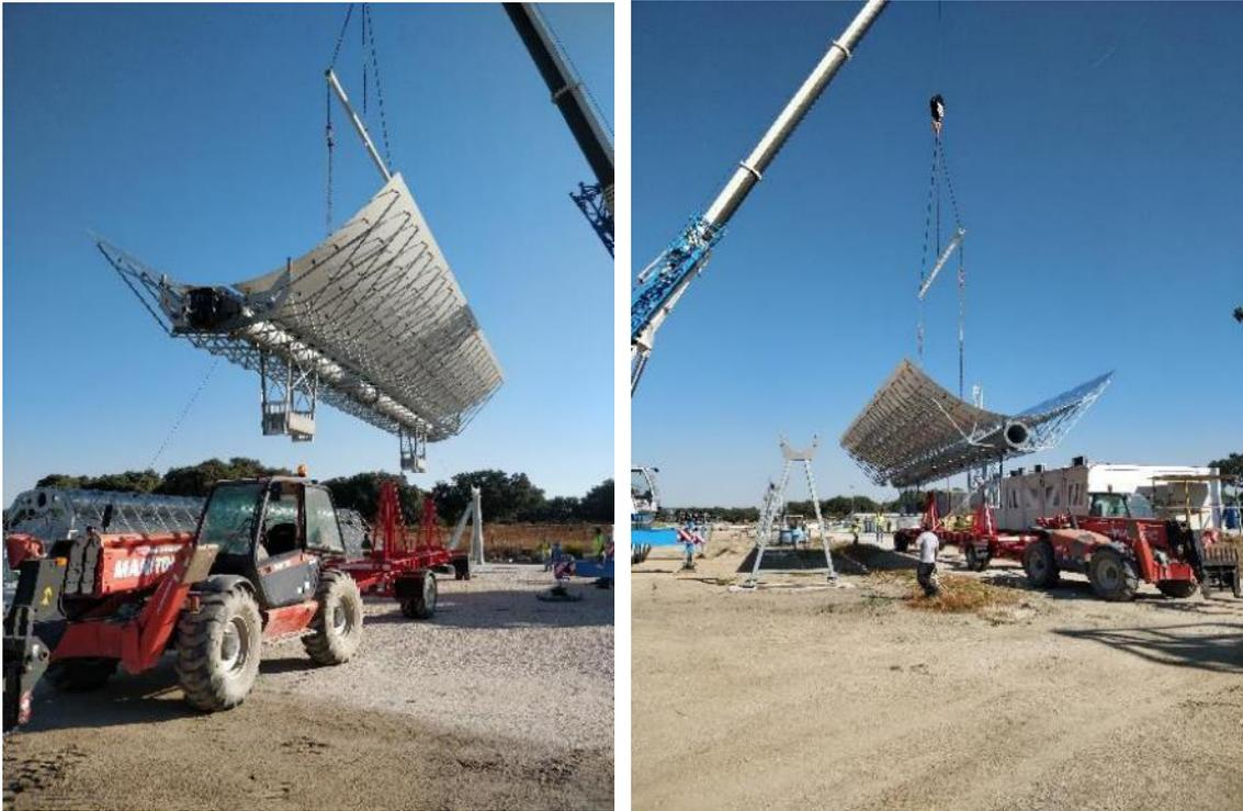
**Figure 37 – Transport of the SCE modules in the field with crane and trailer**
