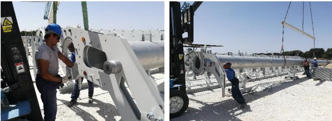
**Figure 28 – Torque Tube assembly and installation of Universal Traverse**
