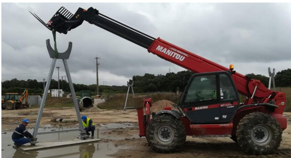
**Figure 20 - Installation of Middle Pylons**
