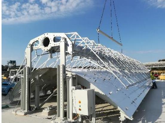
**Figure 32 – Moving the SCE to the Mirror Jig and lower it down with the lifting system**
