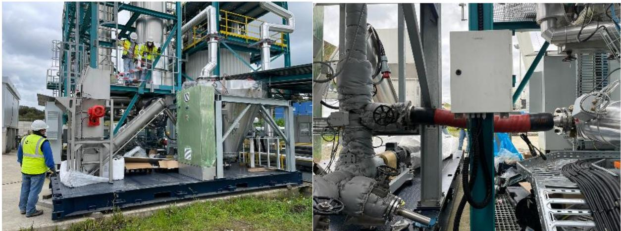
**Figure 2 (Left) Pre-Melting Unit (PMU) installation at EMSP (Right) flexible hose with heat tracing.**
