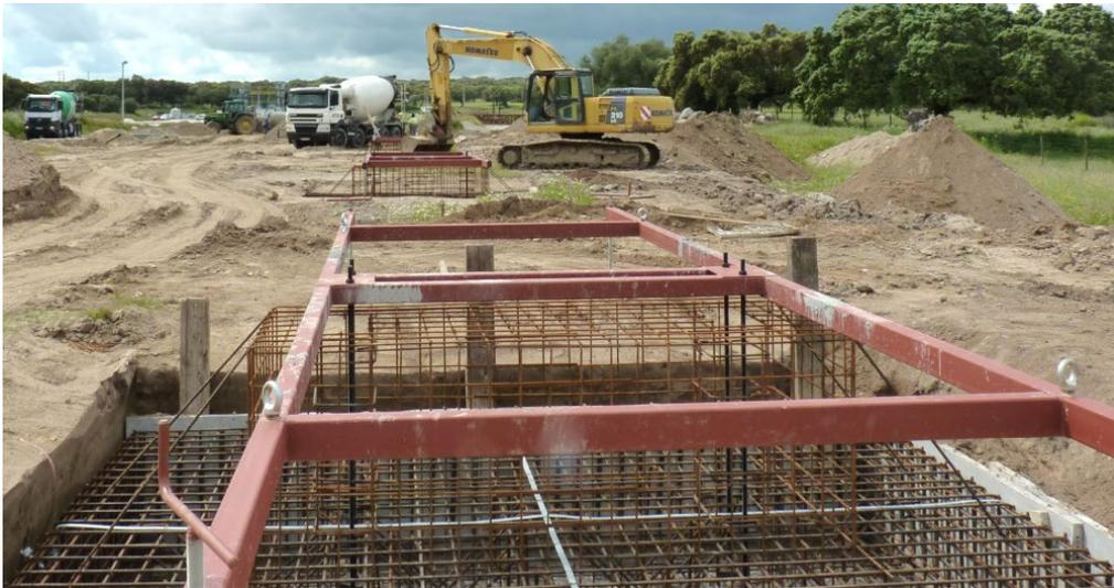
**Figure 18 – Casting of spread foundation base with reinforcements and anchor-bolt templates (red structure)**
