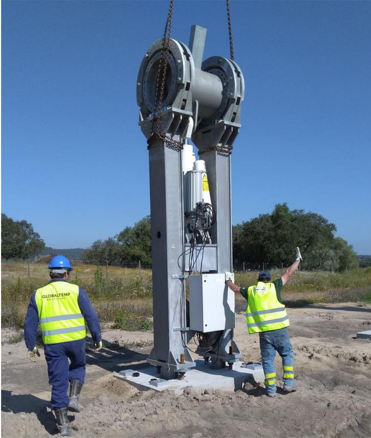
**Figure 21 – Installation of Drive Pylon**
