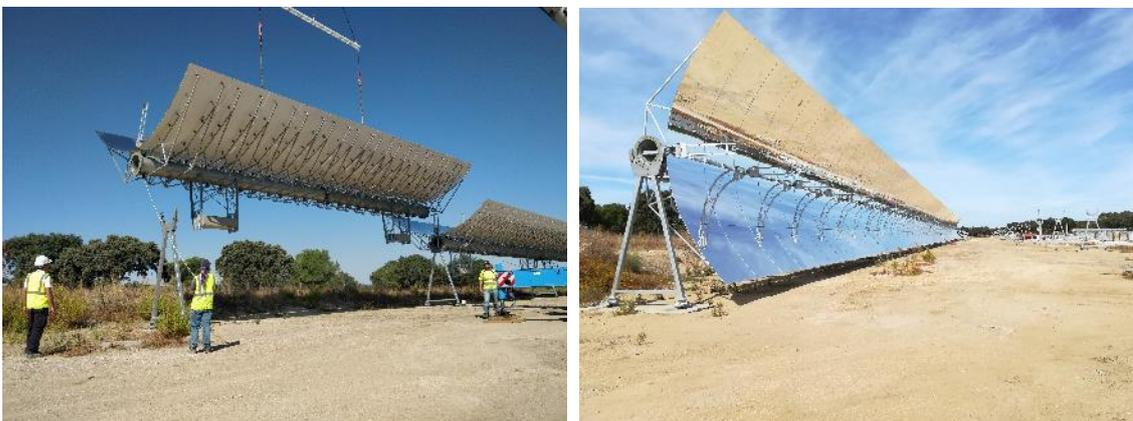
**Figure 38 – SCE modules placed and temporarily fixed in their position**
