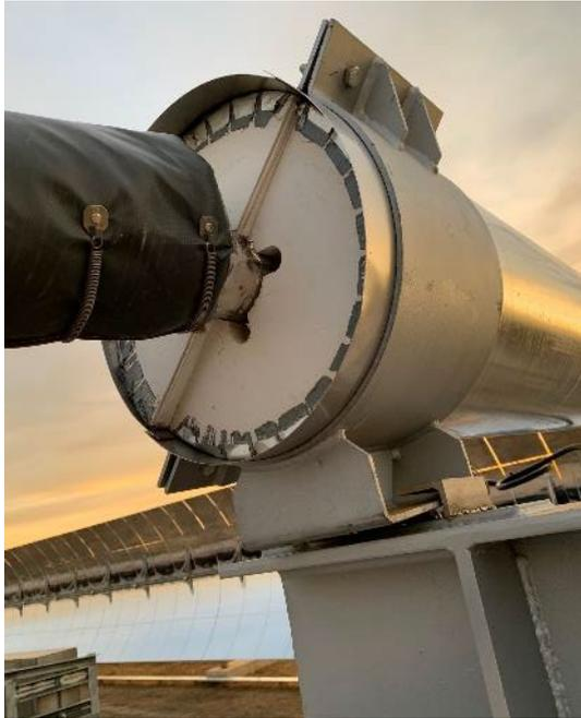
**Figure 84a: Lack of insulation at the COP of the solar field**
