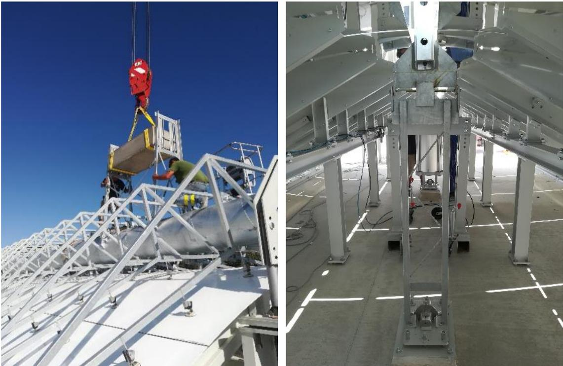
**Figure 34 – Installation of counterweights (left) and HCE-posts (right)**
