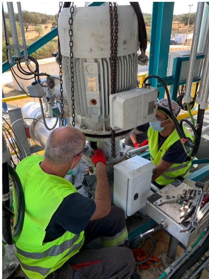
**Figure 64 Maintenance works of salt pump**
