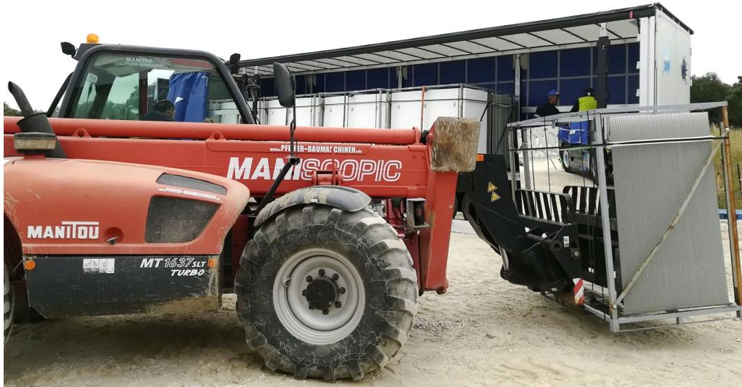
**Figure 13 - RioGlass RP4 mirrors being unloaded on site**
