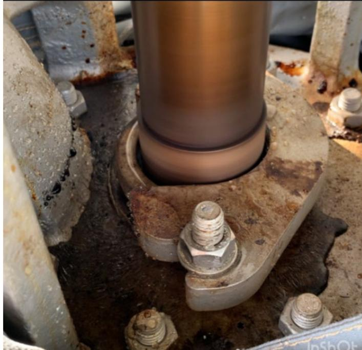
**Figure 78: Leakage of cold salt pump shortly after first start up.**
