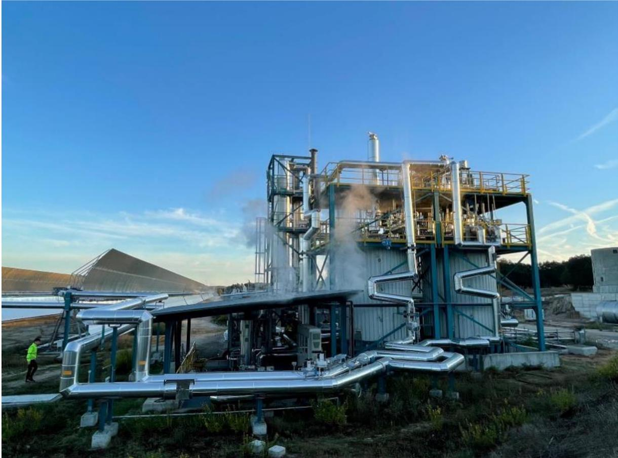
**Figure 3 Steam generation during salt melting**
