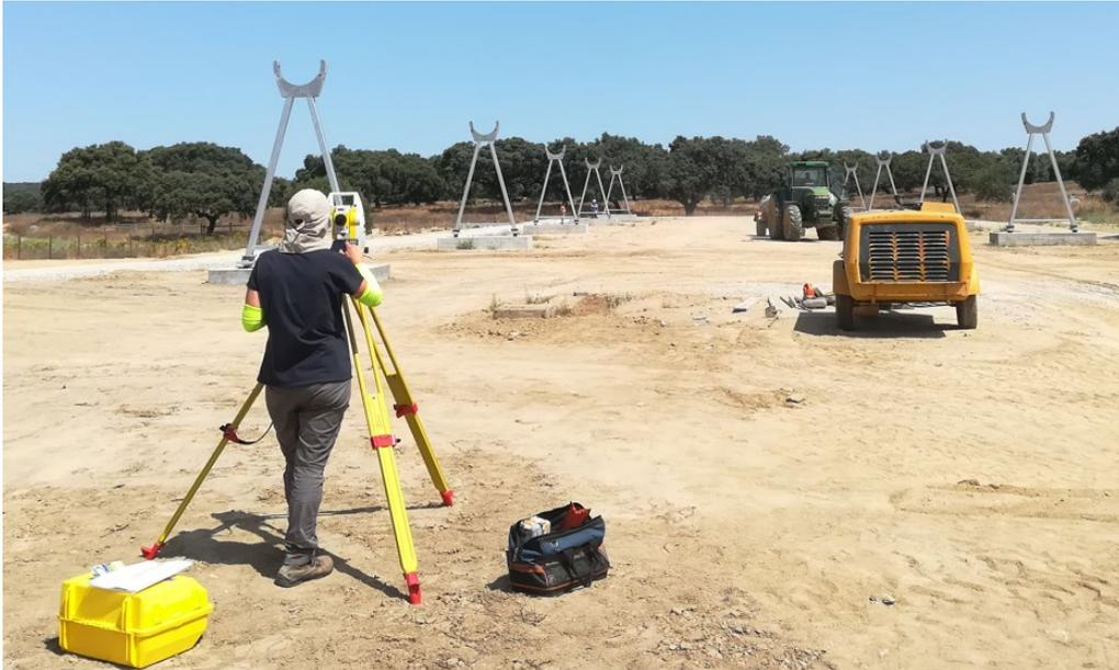
**Figure 22 – Alignment of the Pylons**
