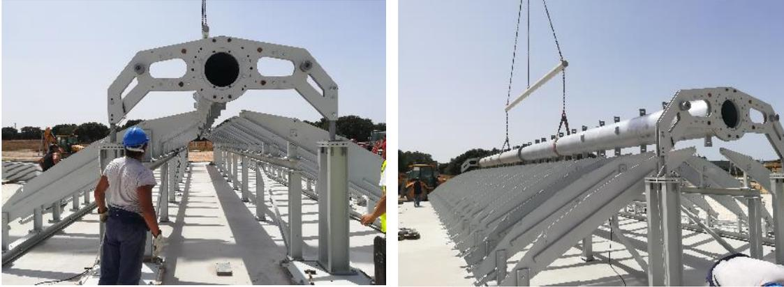
**Figure 29 – TTU flange adjustment in the steel structure Jig**
