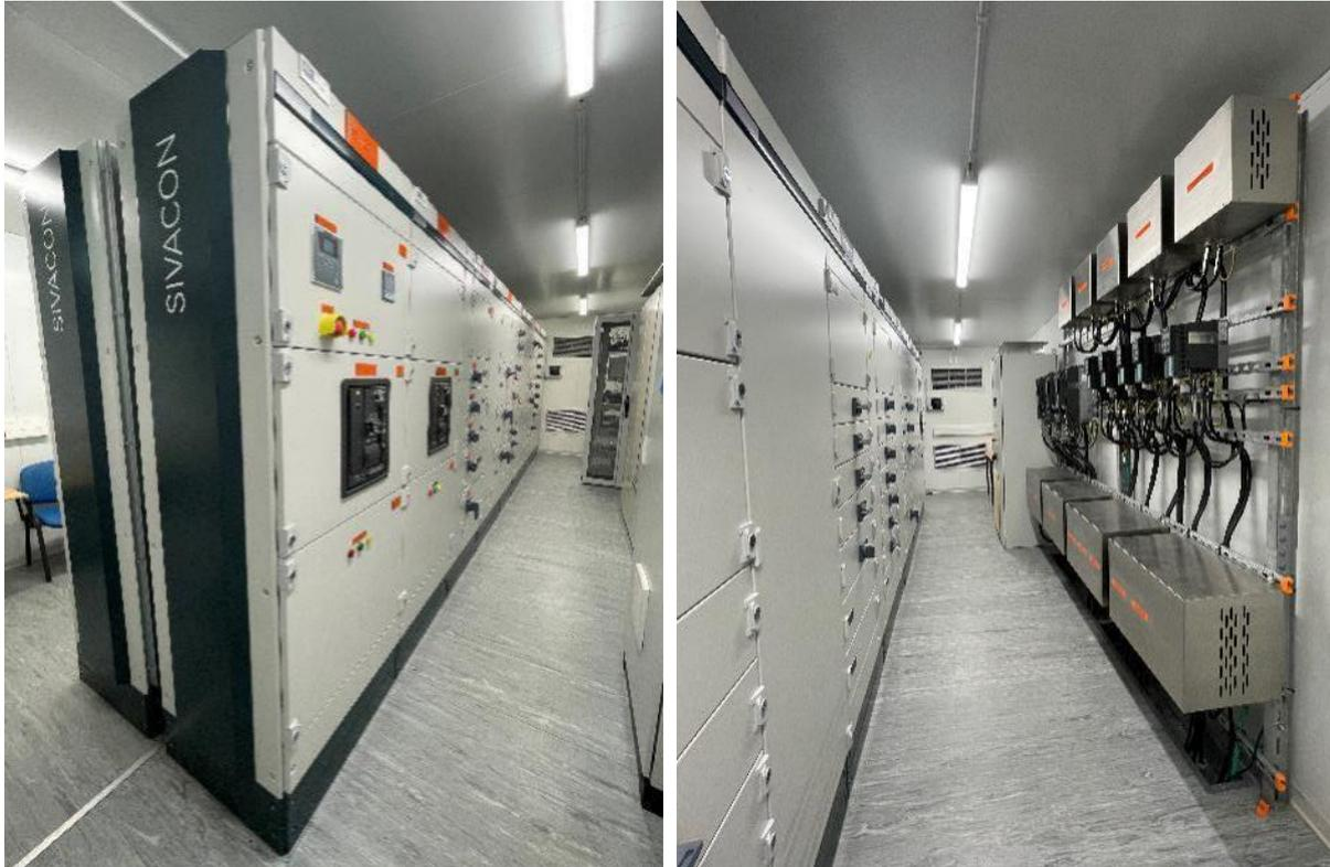
**Figure 63 Photo of the PCC (left) and the MCC (right)**
