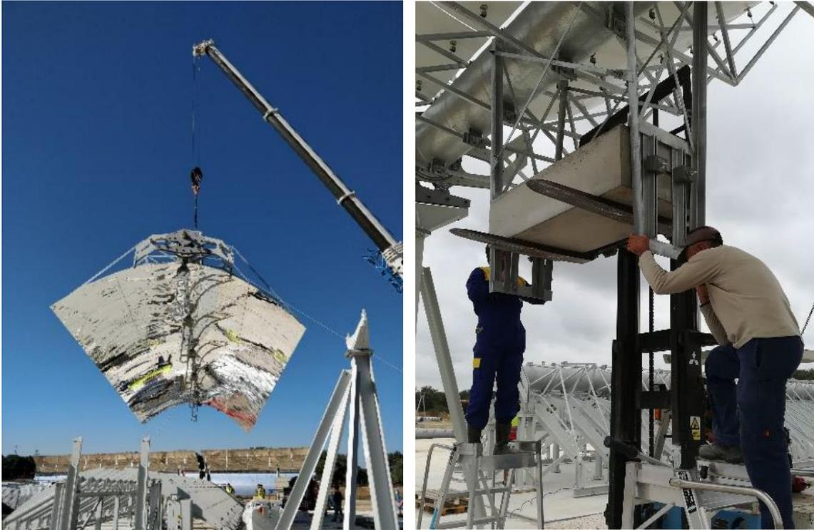
**Figure 35 – Move to the Balancing Station and balancing with Counterweights**
