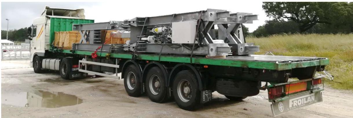
**Figure 15 – Two readily pre-assembled and commissioned drive pylons arriving on site**
