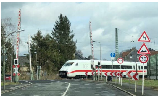
Level crossing fault
