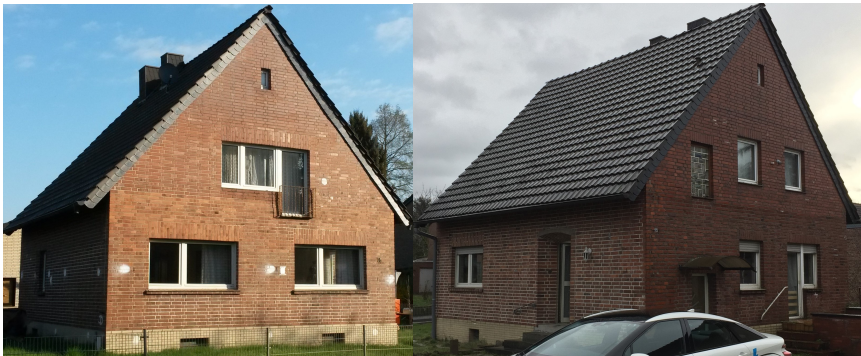
Figure 3.4.: Exterior views on the case study building from a southern (left) and a north-eastern (right) perspective during the preparation of the first and second measurement campaign respectively.
