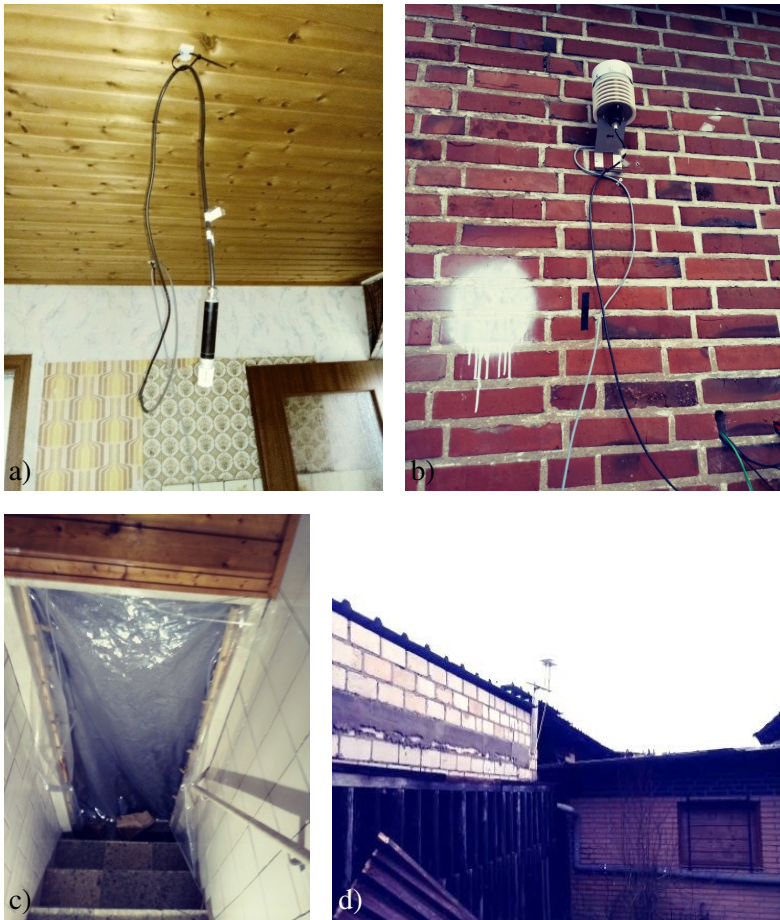
Figure 3.7.: Exemplary parts of the setup for monitoring the conditions during the case study measurement: Temperature sensor in the kitchen (a), combined outdoor sensor for temperature and humidity (b), sealing of the basement entry (c), and solar radiation sensor a few metres off the building (d) [10]. Copyright © 2019 Solar-Institut Jülich der FH Aachen.
