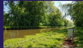
Leakage from canals and reservoirs
