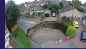
Voids leading to sinkholes
