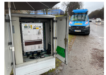
Fig. 5: Intersection control unit to be integrated into the quantum-inspired control system
