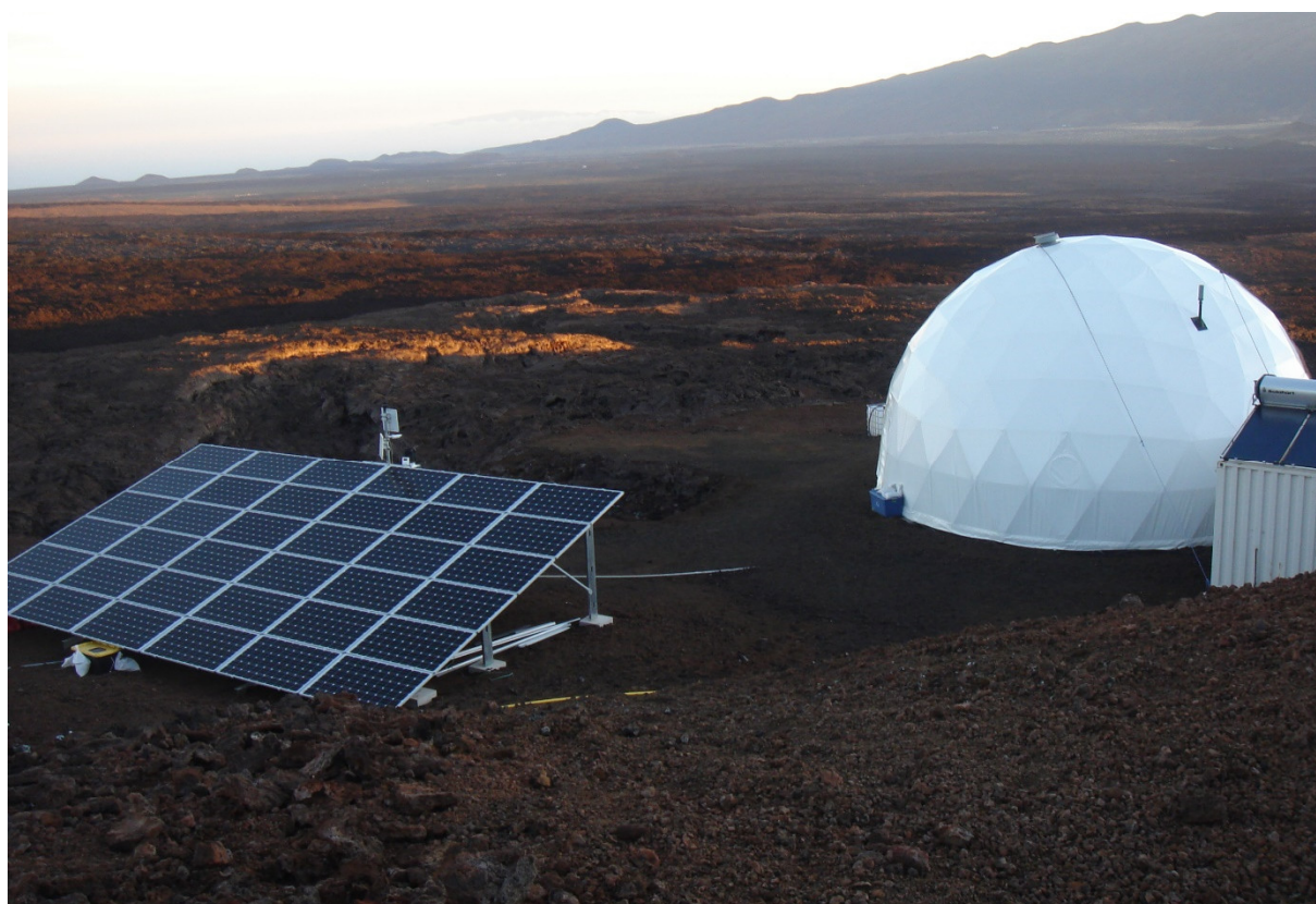
Figure 2.3: HI-SEAS habitat on the slopes of the Mauna Loa volcano. The white dome (center) is attached to a 6.1 m storage container (right) used as a workshop and storage facility. In the foreground (left), solar panels are the habitat's main power source. Photo credits: Lucie Poulet.
