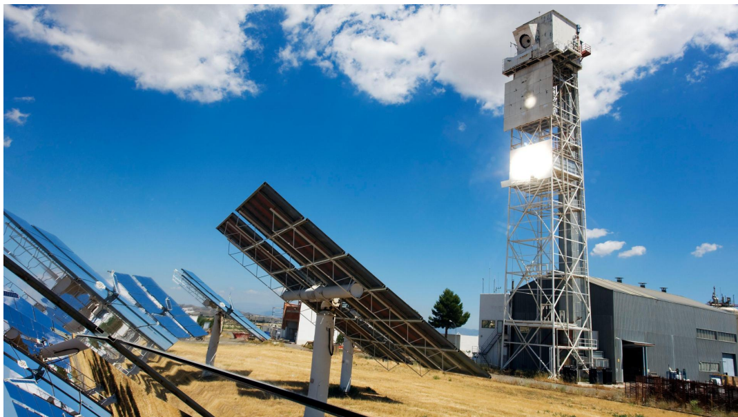
Fig. 1.2.: Solar tower facility at the Plataforma Solar de Almeria, owned and operated by CIEMAT. Heliostats concentrate sunlight on a receiver, reaching high temperatures to drive a power cycle or thermochemical reactions. Source: DLR/Ernsting.
