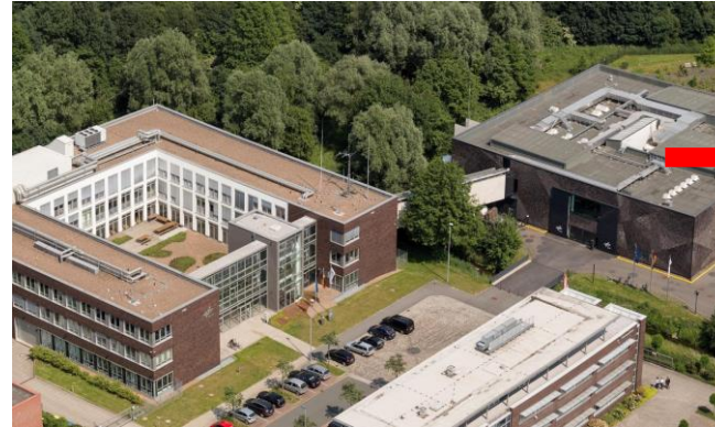
Bremen Maritime Safety and Security Lab
