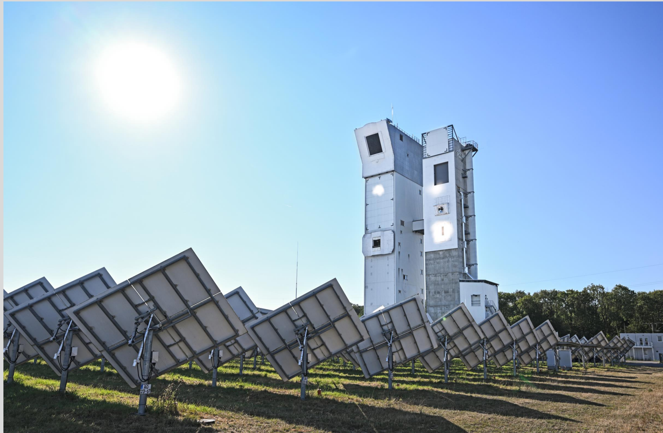
Figure 1: View on the Solar Tower (left) and Multi-Focus Tower (right) in Jülich, Germany. The receiver is irradiated in the middle of the right tower.
