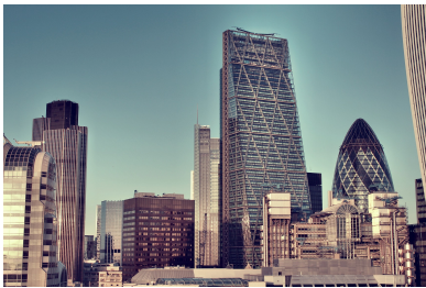
(a) Increase of stiffness by external X-bracing
