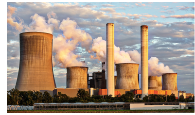
(c) RWE Power plant in Niederaussem, Germany
