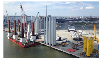
(f) MHI Vestas assembly facility of wind turbines at the Port of Esbjerg, Denmark
