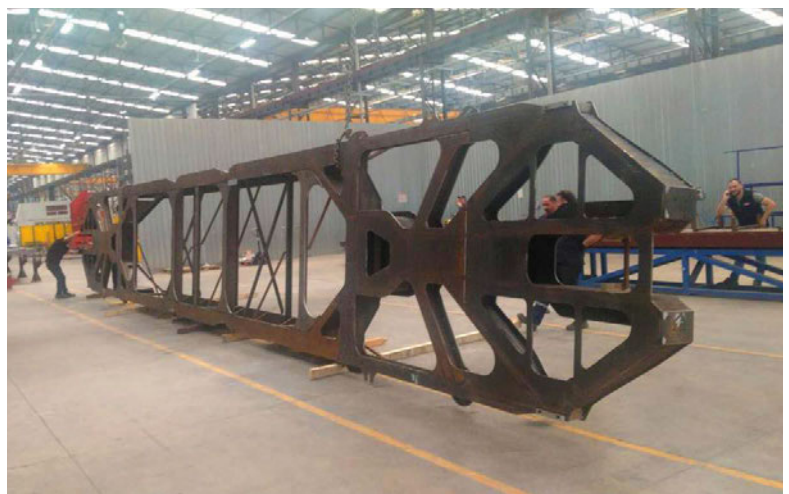
Figure 2 Welded EMW wagon frame being prepared for painting
