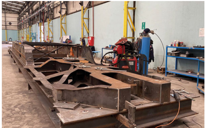
Figure 1 Wagon frame of the EMW during fabrication
