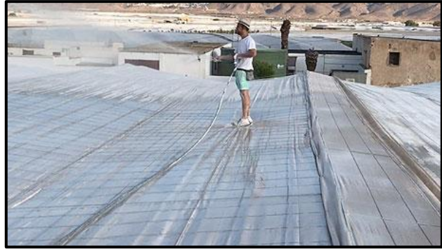
Figure 5: Applying white chalk paint to the roofs of a 'raspa y amagado' greenhouse.
