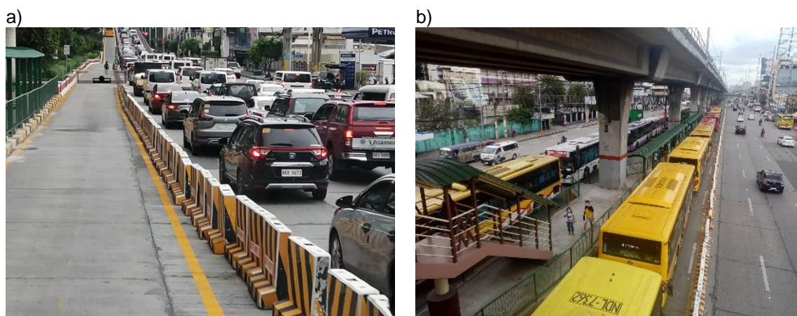
Figure 3.8 (a + b). The newly implemented EDSA Busway BRT in Metro Manila
