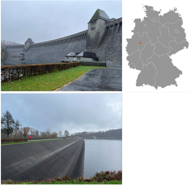
Figure 1: Möhne Dam (top) and Bigge Dam (bottom) as well as their approximate locations in Germany.
